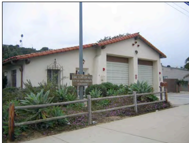
Figure 10 West End of La Cumbre Junior High School City of Santa Barbara Fire Station No. 5
