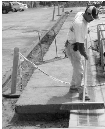
▲ Electrical system replacement at Goleta Valley Junior High
