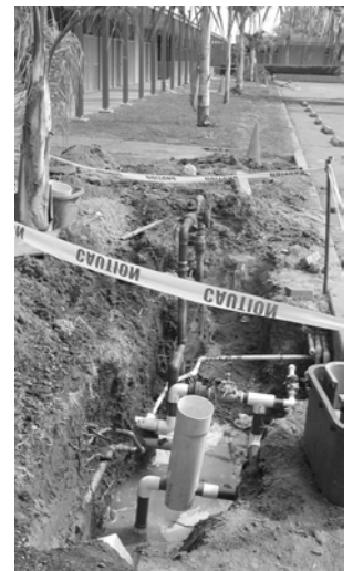
▲ Waterline replacement at Dos Pueblos High School.
